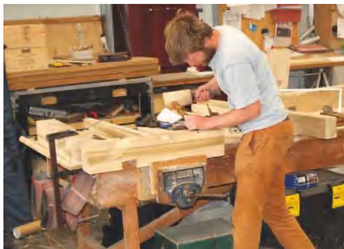
▲ Pic.14 Cutting the housings for the Jack rafters
